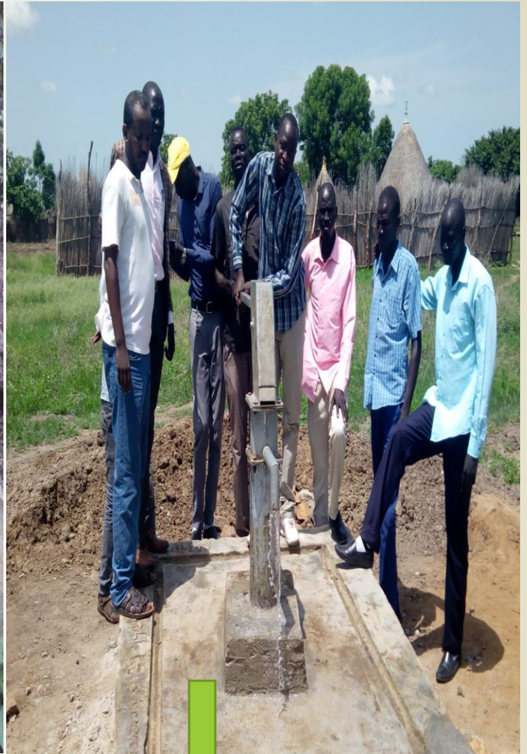
Hand-dug well construction
