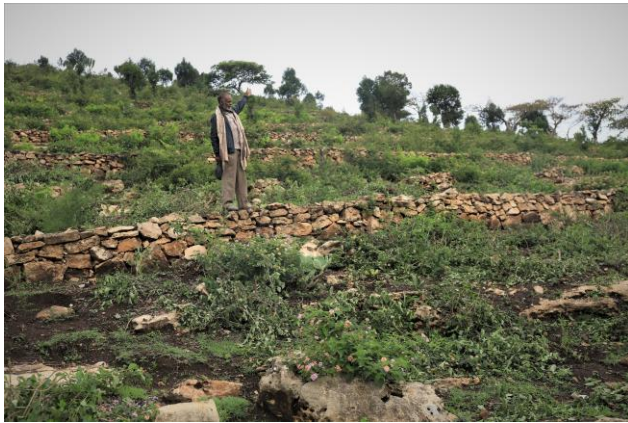
Figure 2 Stone wall bench terrace constructed along the hillside
