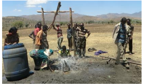
Fig 1. Manual tube well under construction
