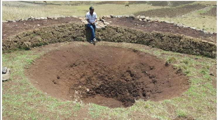
Fig 8. Percolation pit within a shallow waterway with soil embankment and stone paved spillway at the middle
