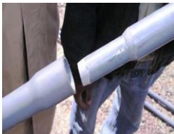
Figure 10.3 – Creating a socket. Heat up the end of the rising main. Insert the tool. Cool the end of the rising main with water (turn the tool around to prevent it from getting stuck). Remove the tool from the rising pipe. The socket is created.
