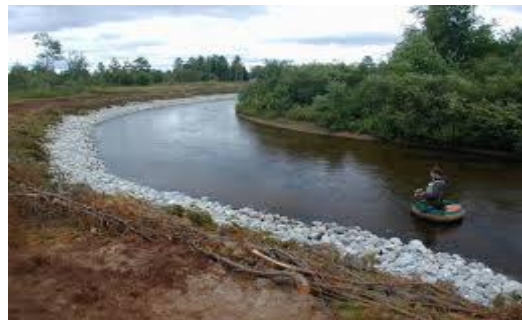
Fig 2. River side stabilization using stone riprap
