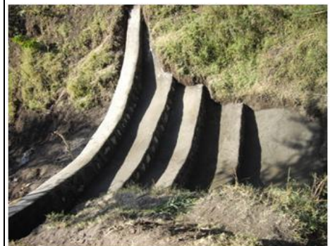
Fig 3. Construction completed Arc-weir checkdam
