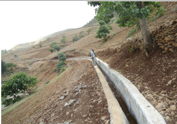
Fig 2. Lined canal laid out along the hillside
