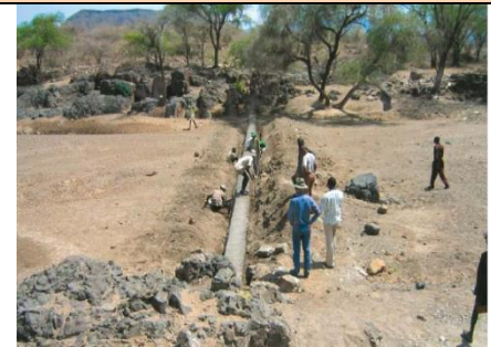
Fig 5. Subsurface dam under construction
