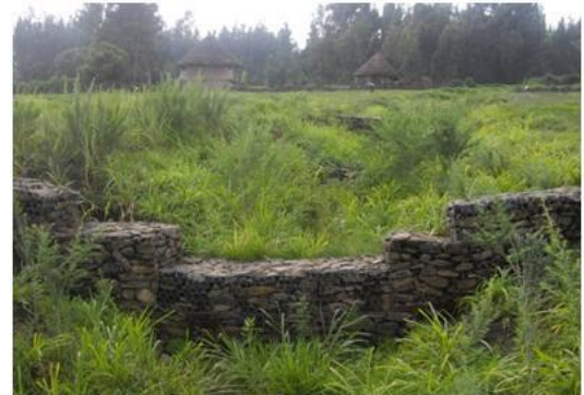
Fig 1. Typical stabilized Gabion check-dam, Farta W.
