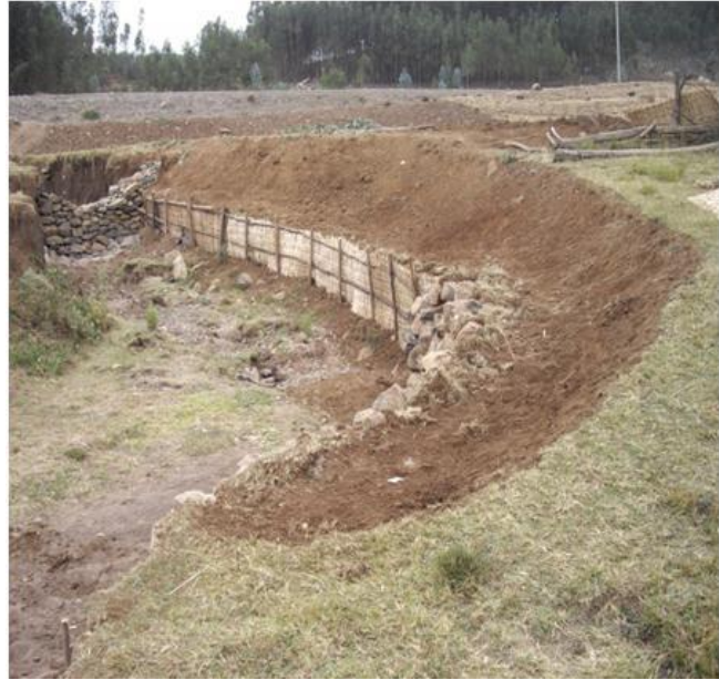
Fig 1. Reshaped Gully with retaining wall
