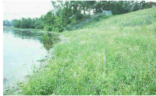
Fig 1. River bank stabilization through vegetation
