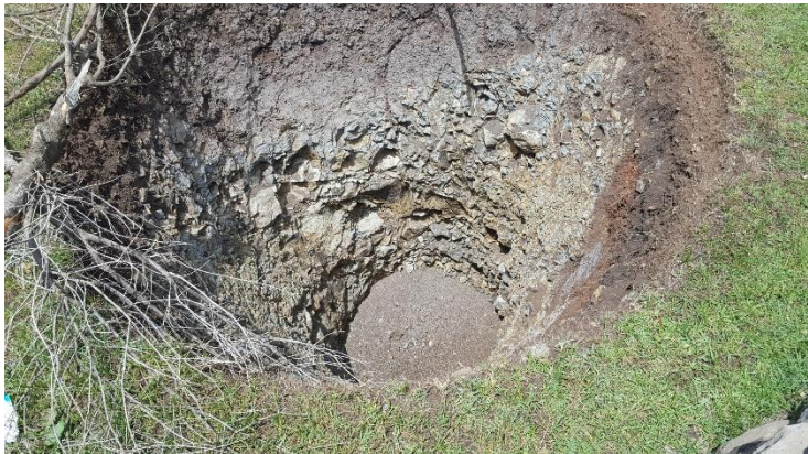
Fig 7. Percolation pit in gravelly soil - cascaded in a waterway
