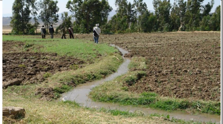
Fig 3. Unlined earth canal drawing water to irrigated fields
