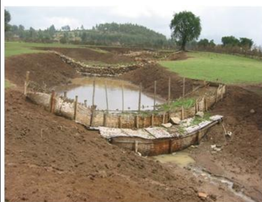
Fig 1. Bamboo-mat checkdam
