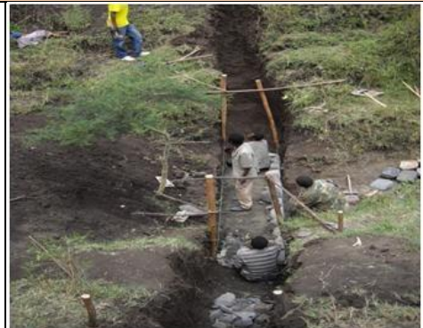
Fig 2. Foundation work for Arc-weir check-dam
