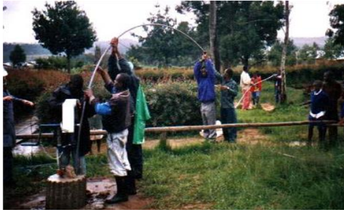
Figure 10.7 Installing the Guide Box with Rising Main and Rope
