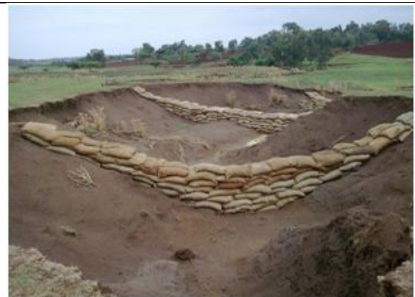
Fig 3. Cascaded sand bag checkdam
