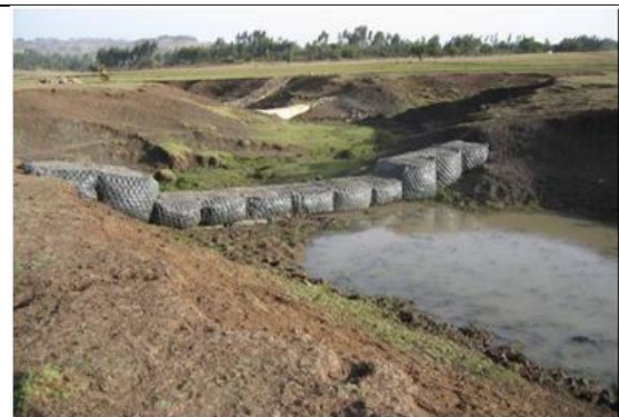
Fig 3. Gabion check-dam construction - soil filled
