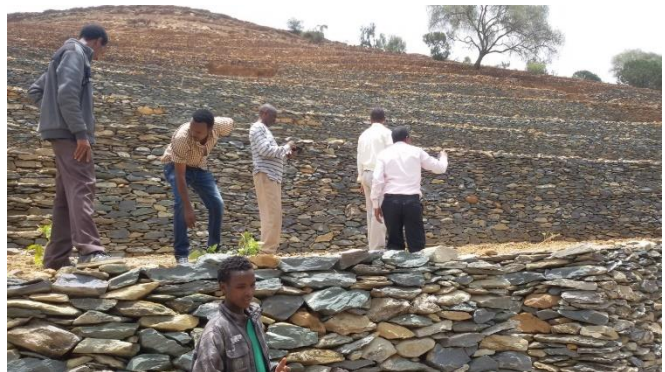
Fig 3. Bench terracing with stone riser under technical evaluation – Tigray, Fereweyni Woreda
