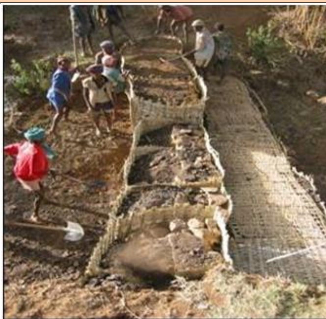
Fig 2. Bamboo-mat checkdam under construction
