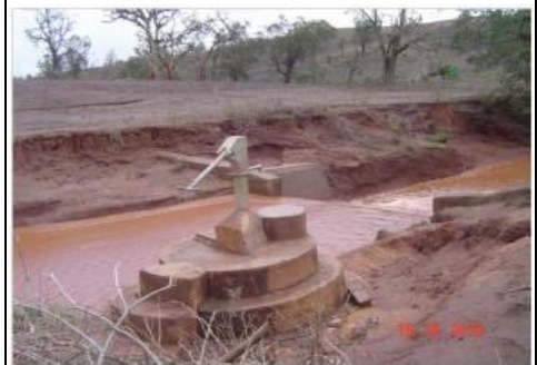
Fig 2. Sand dam with water hand pump close to it for water abstraction
