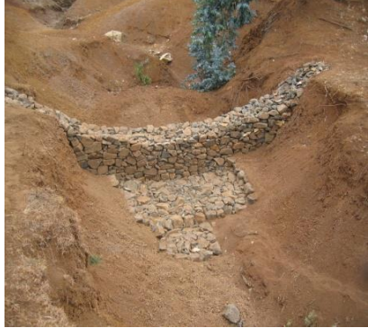
Fig 1. Typical illustration of loose stone check-dams
