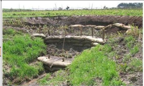
Fig 1. Sand bag checkdam
