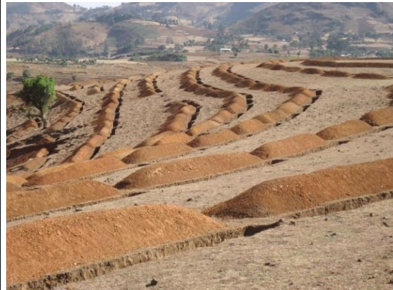
Fig 1. Hillside terracing with trenches, Amhara R., Sekela Woreda
