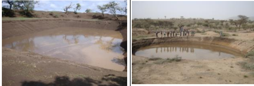
Fig 1. Scene of community ponds (trapezoidal – left) and circular (right) in dry areas primarily for LS purpose
