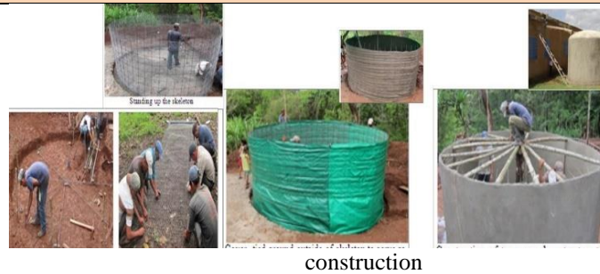
Fig 3. Different stages of tank under construction
