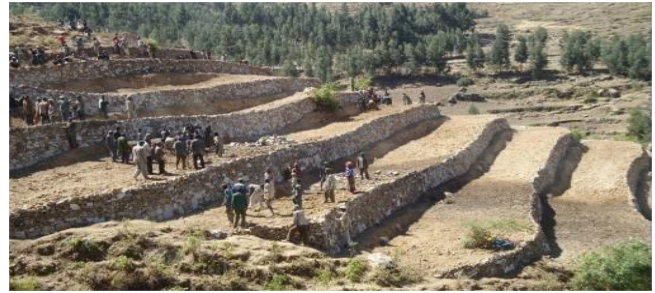
Fig 1. Bench terrace under construction, Meket Woreda
