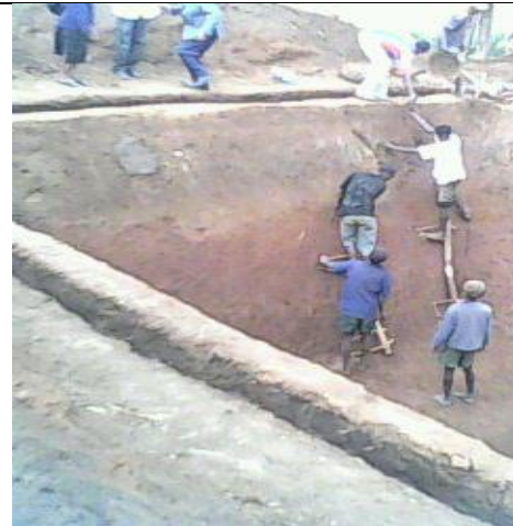
Fig 4. Elimination of the steps and final shaping of the pond
