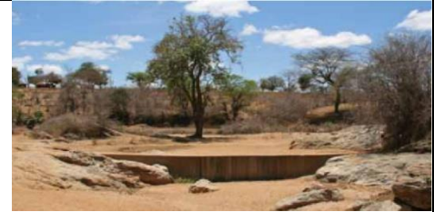
Fig 1. Sand dam in dry river
