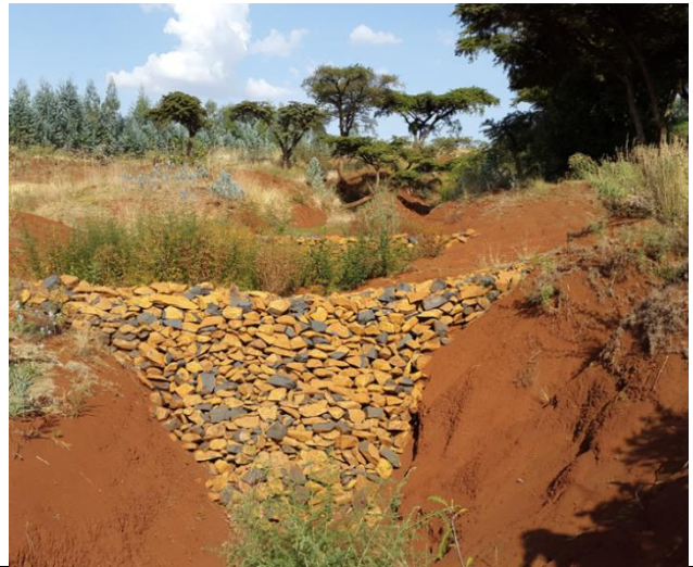
Fig 1. Sediment storage dam
