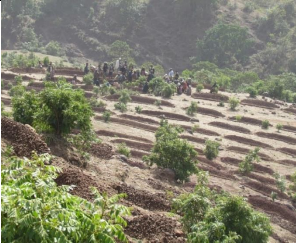
Fig 5. Trenches for groundwater recharging, staggered, Amhara R., Dera Woreda
