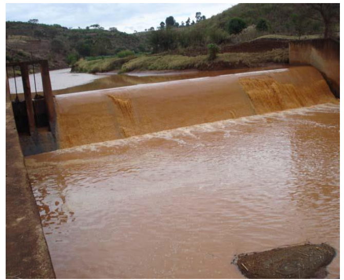
Fig 5. Diversion weir functioning, see the control gate (left)
