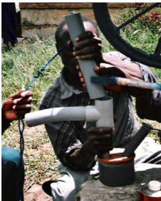
Figure 10.8 Connecting PVC Pipes
