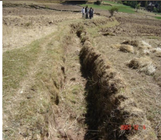
Fig 1. A well-established grassed cutoff drain
