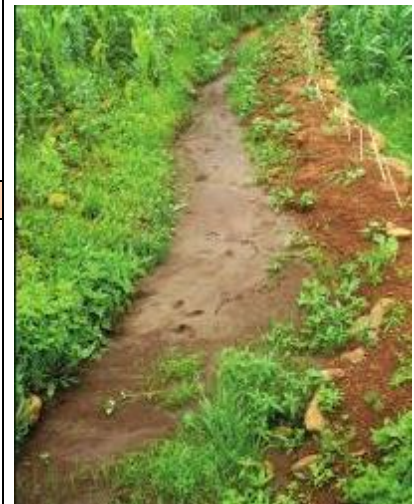
Fig 1. Graded soil bund, water flowing towards the viewer
