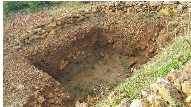
Fig 2. Function of percolation ponds in the capturing of silts. See the flood mark from the side of the inner pond and feel the water that has soaked instead of being lost as runoff .
