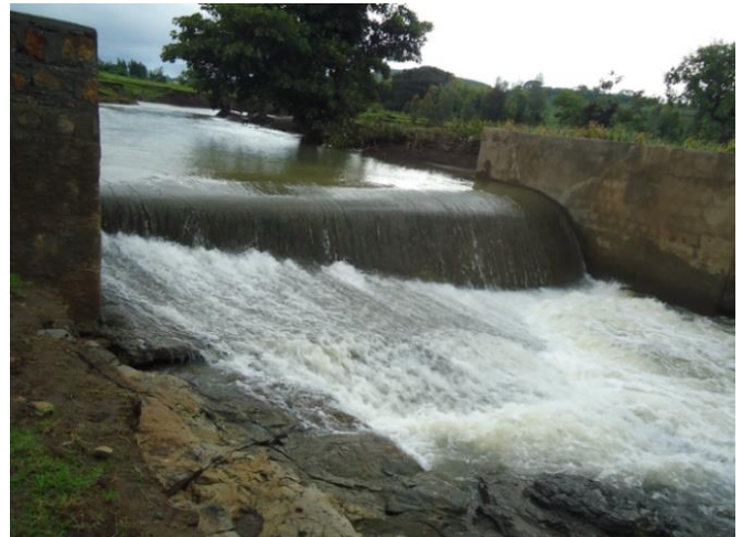
Fig 7. Upstream and downstream scene of the weir structure
