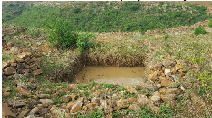
Fig 1. Function of percolation ponds in capturing runoff and recharging of the groundwater to later be used as springs, streams and hand dug wells.
