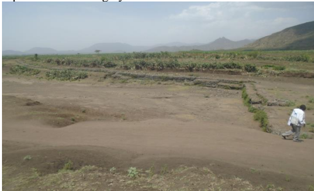
Fig 2. Gabion diversion structure
