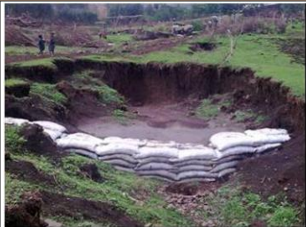
Fig 2. Sand bag checkdam ready for gully side reshaping
