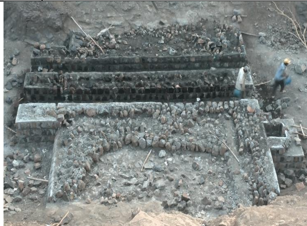
Fig 5. Double silt excluder
