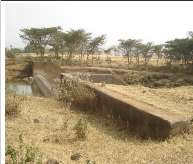
Fig 4. Scene of a diversion weir
