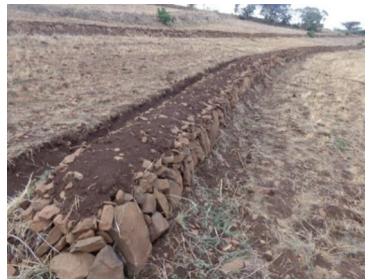
Figure 46: Stone-faced soil bunds constructed on farmland (Ejere woreda, Gunjo, Oromia).
