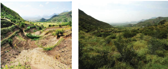
Figure 102: Restored gully (Raya Azebo woreda, Tigray).
