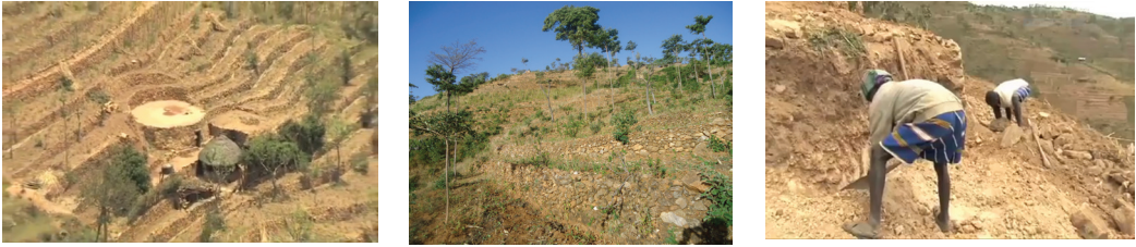
Figure 1: Construction of soil and water conservation terraces by a Konso community.
