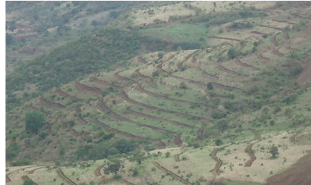
Figure 52: Hillside terraces constructed with soil (Ambo woreda, Oromia).
