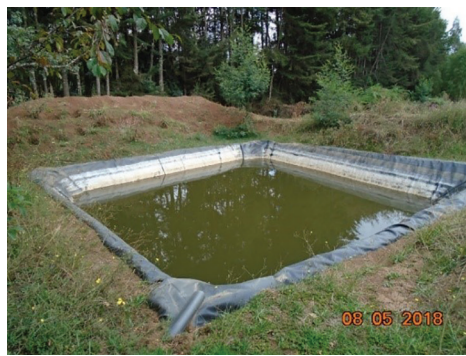
Figure 72: Household-level pond constructed with geo-membrane (Amhara).
