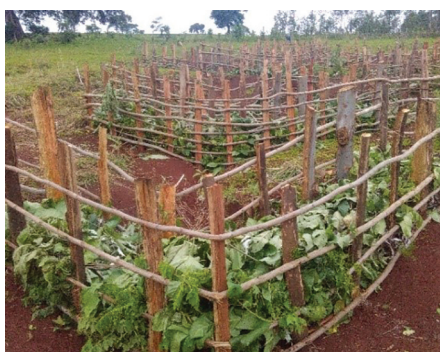
Figure 63: Check dam constructed with brush wood (Hawa Gelan woreda, Oromia).
