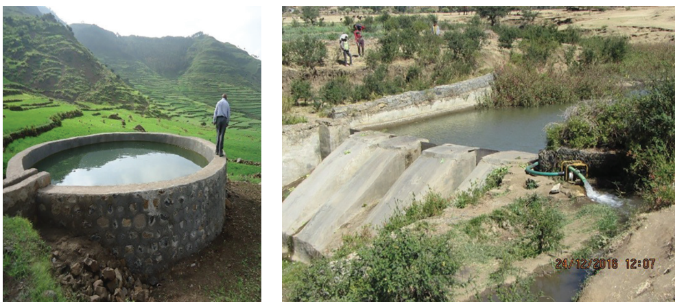
Figure 128: Partial view of storage structures established in SLMP watersheds. Source: GIZ SLM archive, 2020 - Tigray region.
