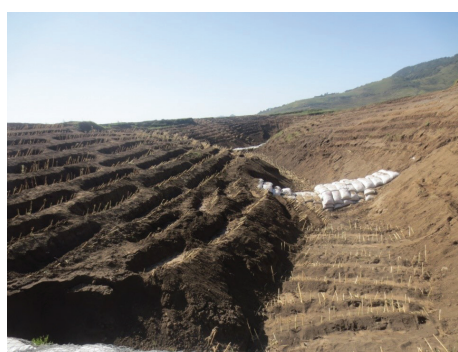
Figure 64: Check dam constructed with sandbags (Endamkoni woreda, Tigray).
