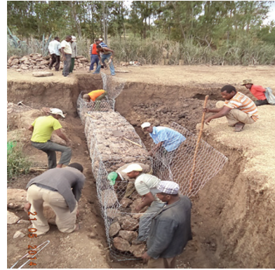
Figure 60: Community constructing gabion check dam across a gully (Lume woreda, Oromia).
