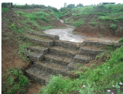
Figure 70: Gully changed to productive land due to sediment storage dam construction (Lume woreda, Oromia).
