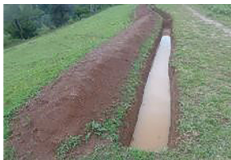
Figure 44: Level soil bund with tie ridge and collected rainwater (Jmma, Ambo, Oromia).
