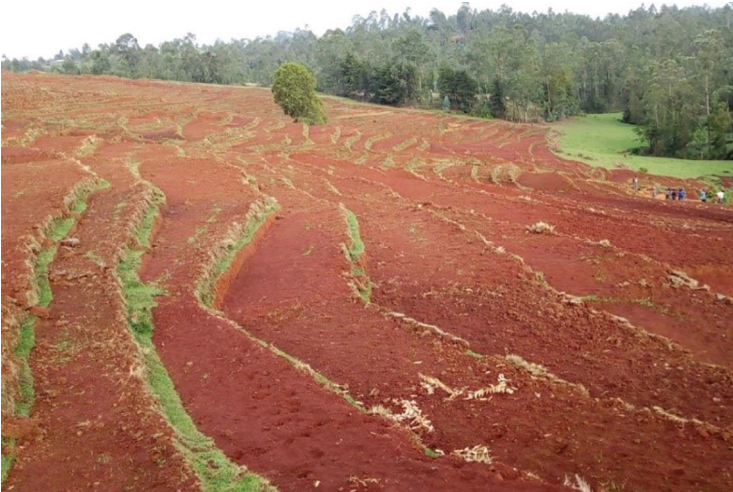
Figure 55: Bench terraces constructed by earth cutting (Gumer woreda, SNNPR).
