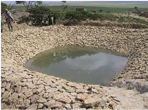
Figure 71: Household-level pond constructed from stone.
