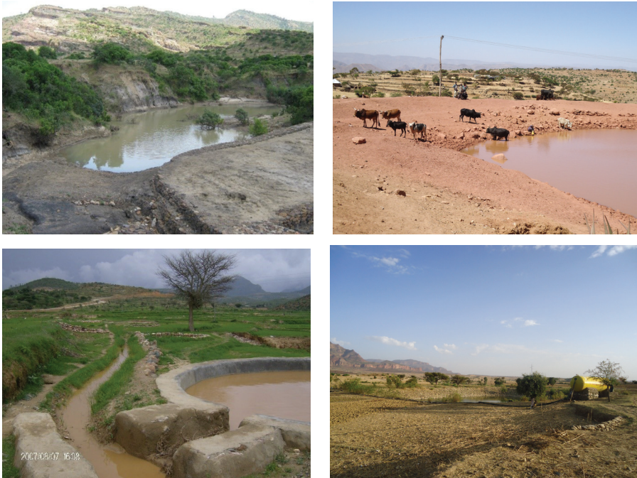
Figure 5: Watershed collection ponds constructed for reforestation and livestock watering in Tigray.
