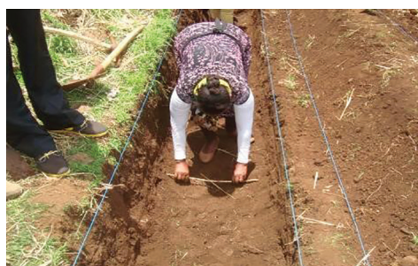
Figure 43: Constructing soil bund and measuring dimensions for quality management (Ade'aBerga, Oromia).
