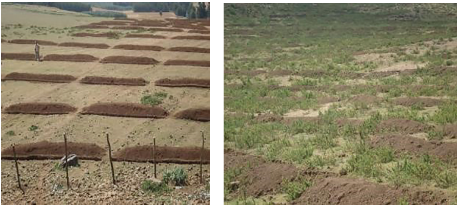
Figure 57: Trench construction on degraded grazing land (Sinan woreda, Amhara).
