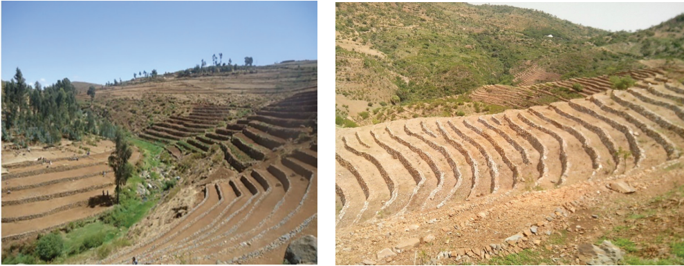
Figure 54: Bench terraces constructed from stone on hillside area in Atsbi Wonberta watershed (left) and Sheka micro-watershed (right), Tigray.
