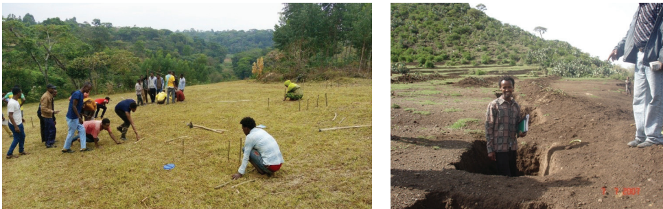
Figure 32: Trained field technicians making contour lines before the construction of a soil and water conservation structure (left) and measuring the depth and width of the structure after construction (right).
