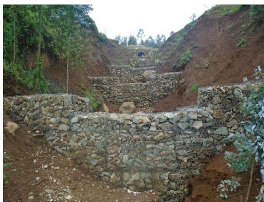
Figure 184: Gabion wires used for check dam construction in Amhara.
