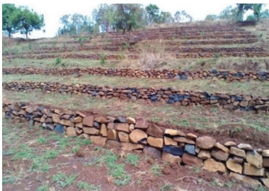
Figure 51: Hillside terraces constructed with stone (Hawa Gelan woreda, Oromia).
