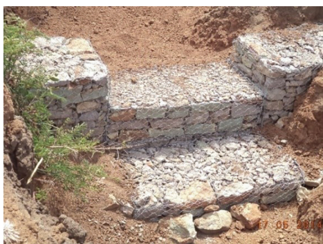
Figure 61: Check dam constructed with gabions (Lume woreda, Oromia).
