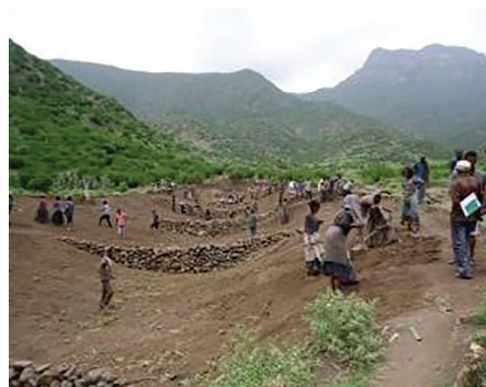
Figure 62: Check dam constructed with loose stone (Raya Azebo, Tigray).
