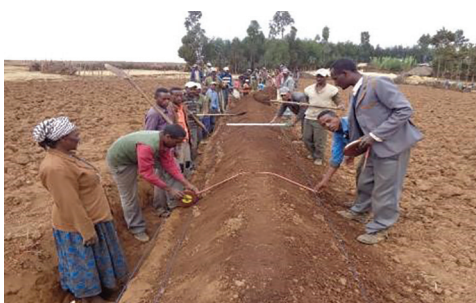
Figure 43: Constructing soil bund and measuring dimensions for quality management (Ade'aBerga, Oromia).
