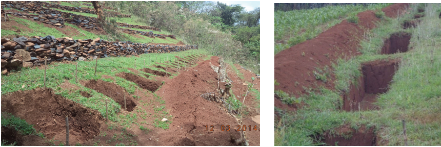
Figure 56: Trenches with hillside terraces (Alle woreda, Oromia) (left) and: deep trench on farmland upper catchment (Ana Sora woreda, Oromia) (right).
