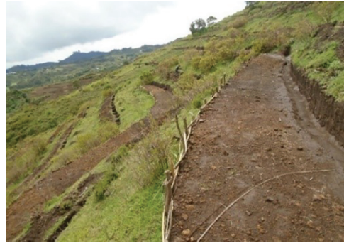
Figure 50: Hillside terraces constructed with bamboo (Wonchi woreda, Oromia).
