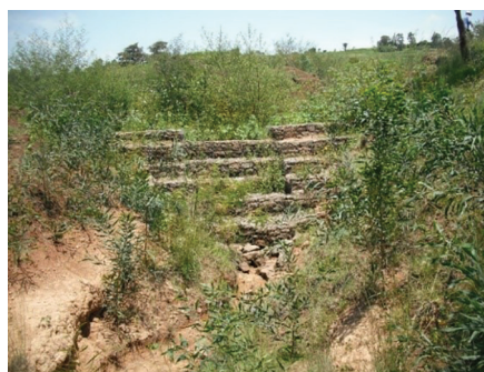
Figure 70: Gully changed to productive land due to sediment storage dam construction (Lume woreda, Oromia).
